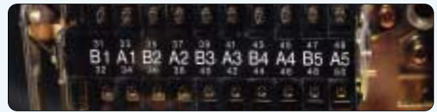
[ Auxiliary switch assembly ]
